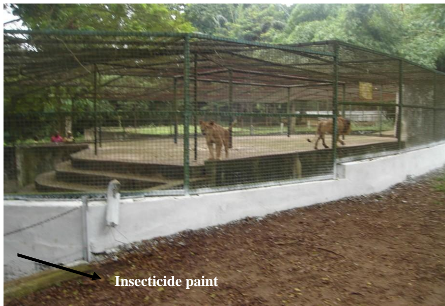
Fig. 2. Insecticide paint applied to the wall in the cage of lions
